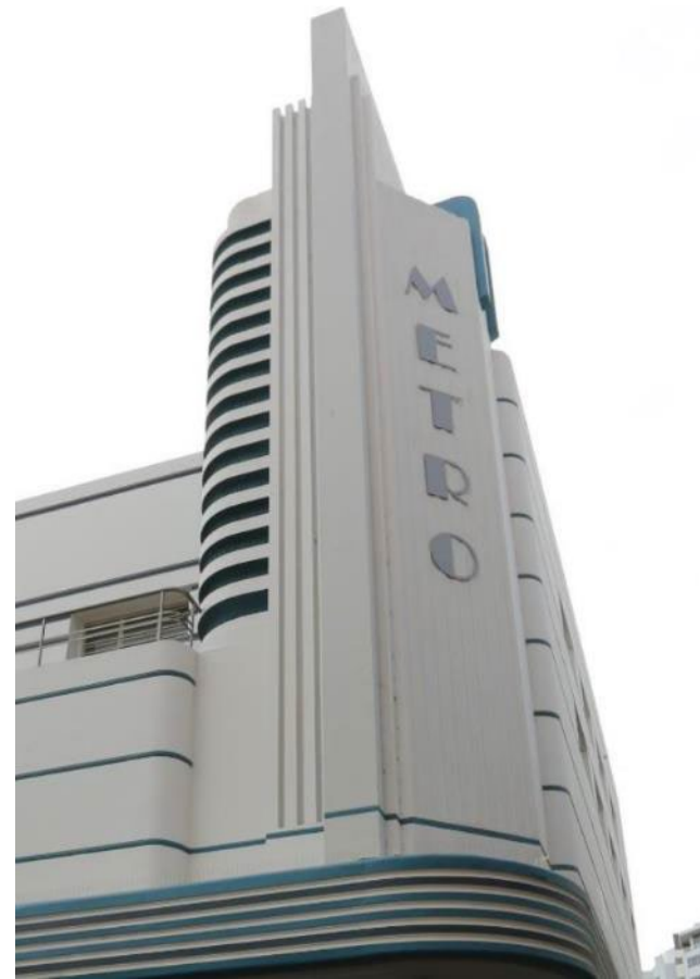
fly tower and corner feature
